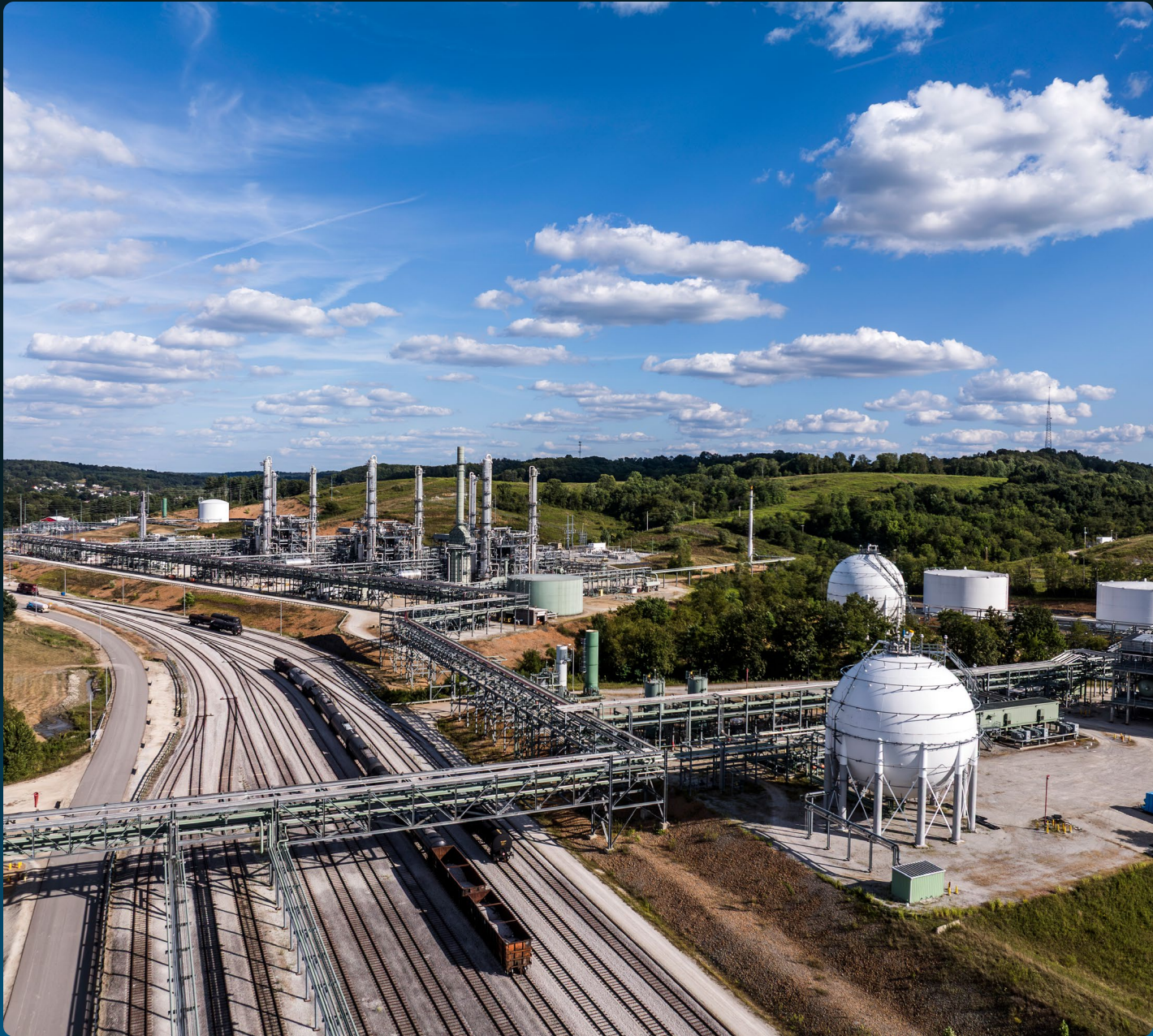
Harrison Hub Gas Processing Plant near Scio, Ohio.
