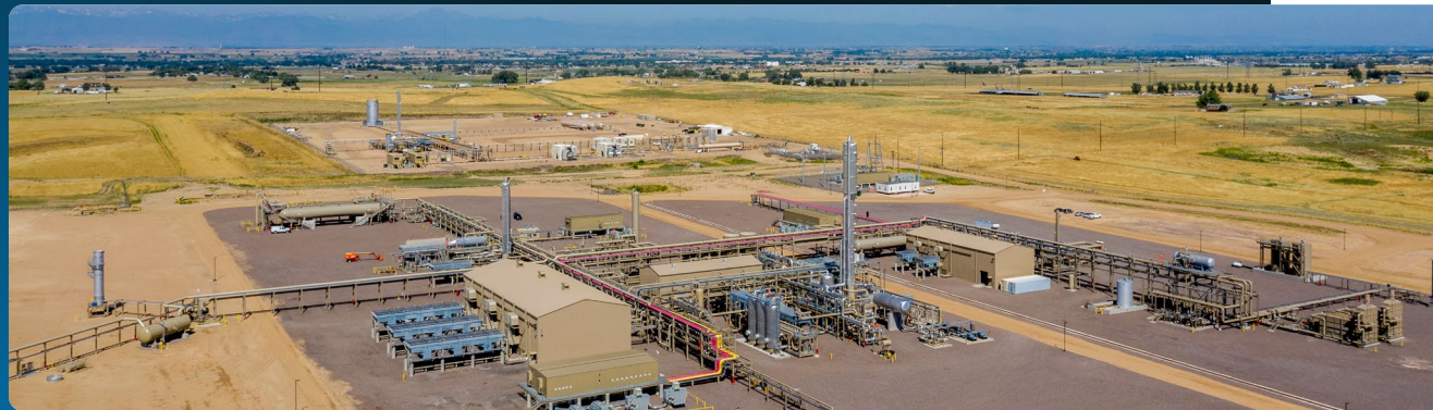
The Fort Lupton Gas Plant near Fort Lupton, Colorado.
